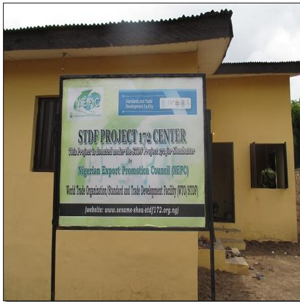
STDF building in Saki Town
